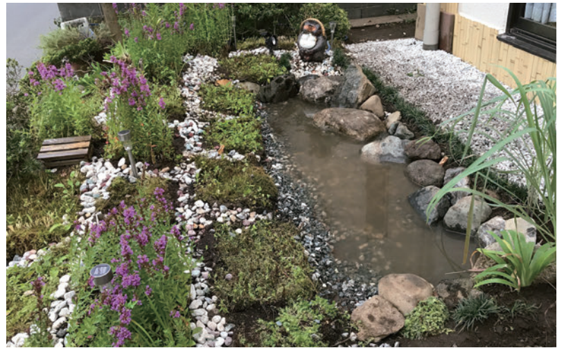
Site-1 Iwase Community Center "Japanese style rain garden"
